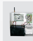
POWER SUPPLY BACKUP BATT BOX
